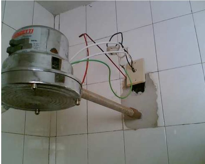
Figure 35: Typical electric shower in a Brazilian household
