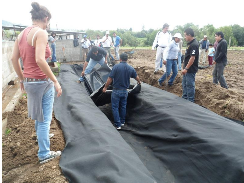
Figure 18 The bag-type biodigester is placed inside the ditch
