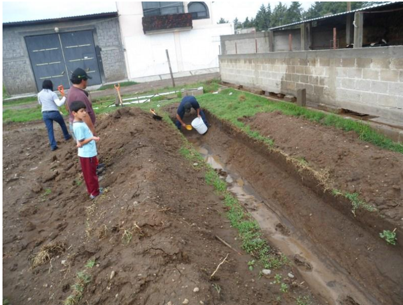
Figure 16 Pitch ready for biodigester installation
