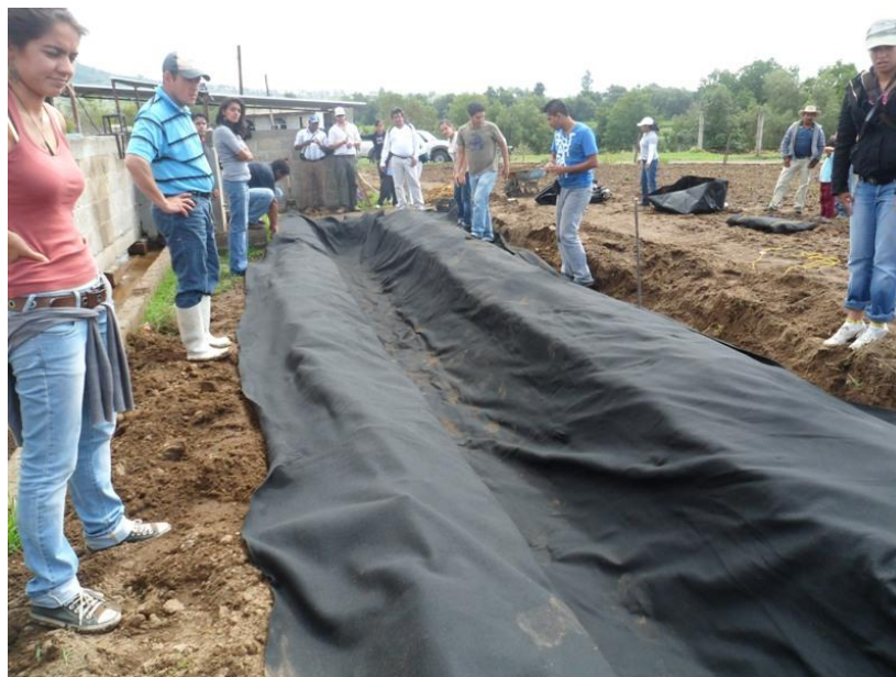
Figure 17 The geotextile liner is placed on top of the ditch
