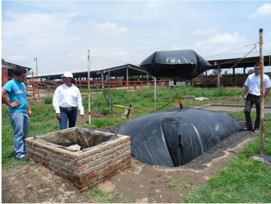
Figure 12 Functioning biobolsa system located in Tlaxcala, Mexico
