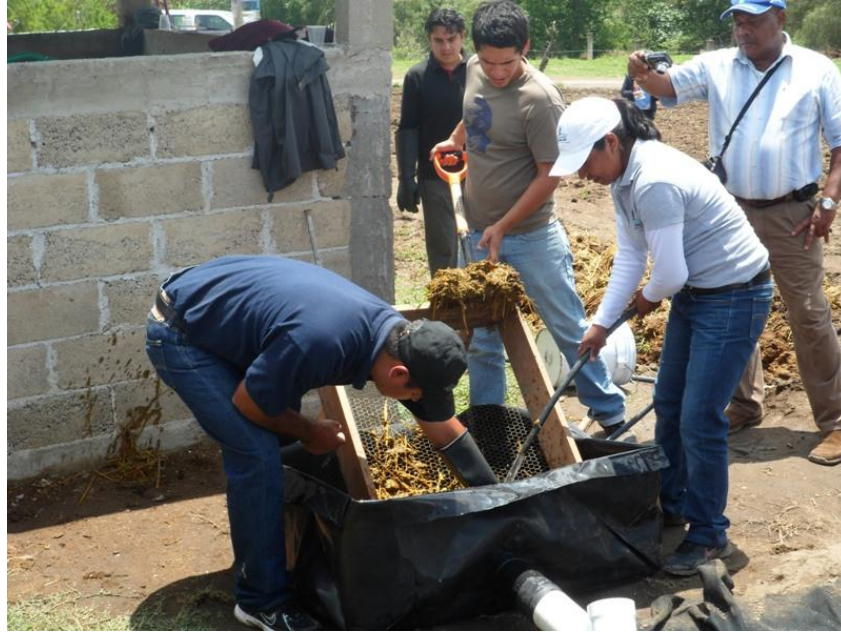
Figure 20 Manure loading to the biodigester
