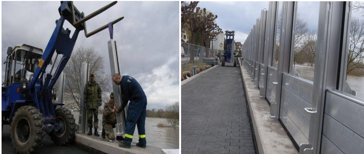
Figure 40 – Temporary flood walls being installed next to the Rhein River. Source: SteB, 2012.
