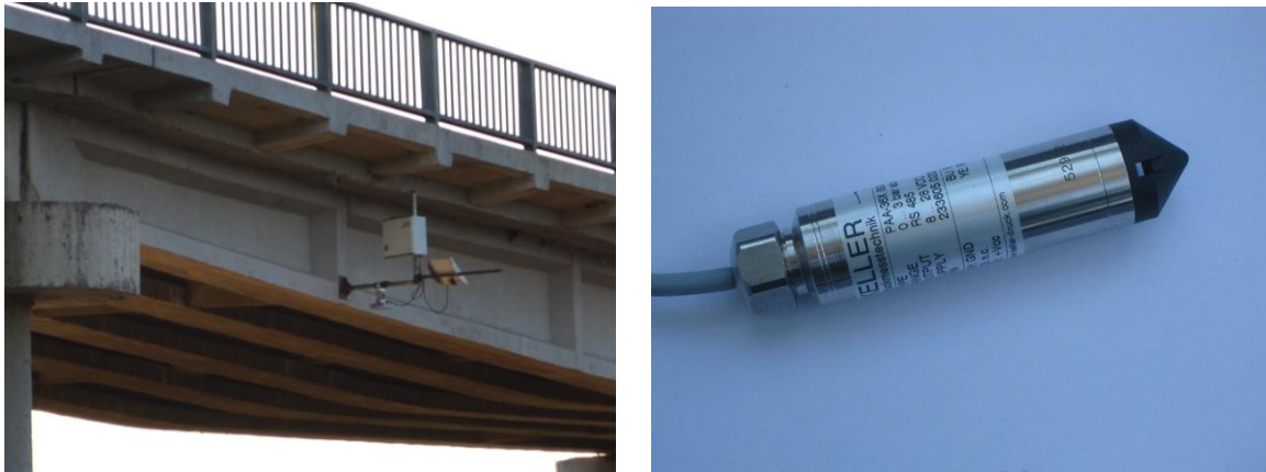
Figure 33 - Example of a radar station and a pressure sensor respectively.
