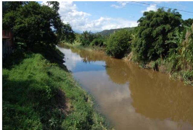
Figure 18: Typical aspect of lowland sections of the rivers where channelization has been executed. Notice the steep banks. In this case Guapiaçu river at the assessment point "06_GAC".
