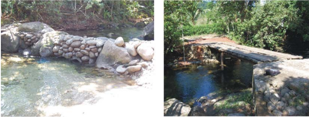
Figure 17: Examples of the most frequent disturbances to stream channel found in upstream reaches: small dams made of rocks and bridge abutments. These two are from Caboclo river at the "07_CABA" point.
