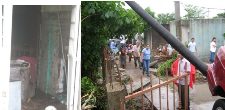
Image 37 Internal household damage (left), damaged furniture (chairs) (right).
