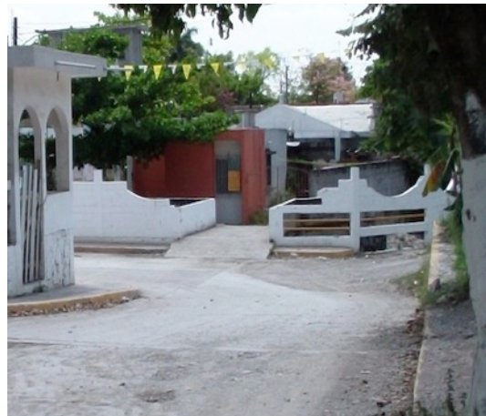
Image 24 Adjustment of protection wall in order to discharge overflow from streets back to the river channel. Source: own
