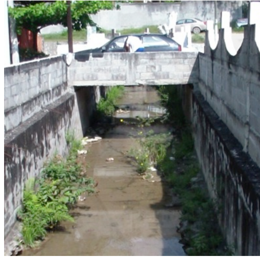
Image 17 Reinforcement of the channel, made by neighbors with help of City Hall. Source: own
