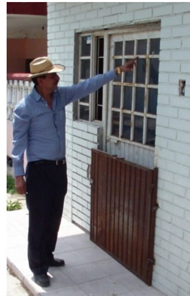
Image 7 Specialized informant shows the flood level reached in 2008, evidenced by the rusty metal at the door. Source: own
