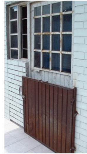
Image 27 Household-level infrastructure adjustment at Magisterial suburb: Metal protection for doors. Source: own
