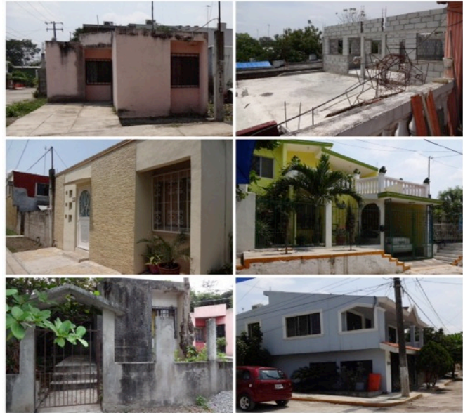
Image 26 Physical adjustments at household-level infrastructure at Magisterial suburb. Top left photo shows original design of households (according to specialized informant), top right photo construction of second floor of house. Photos from the bottom example of diverse adjustments. Source: own
