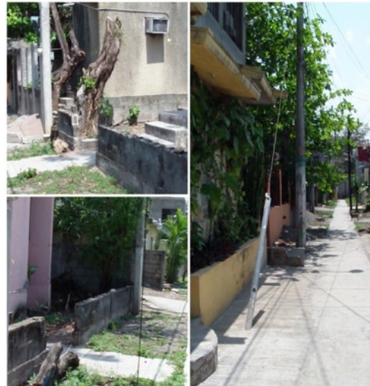
Image 16 Shared design on houses' entrance with a stone fences to protect house from flood impact. Source: own
