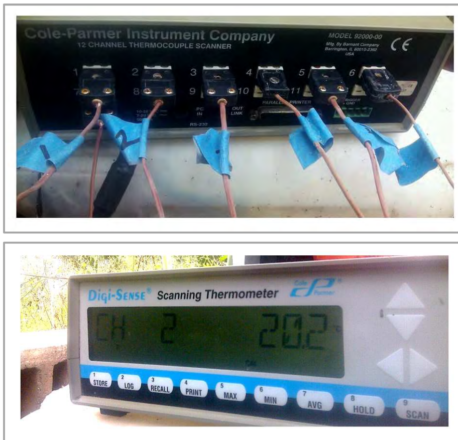
Figure 39. Thermocouples for subsoil temperature measurements
