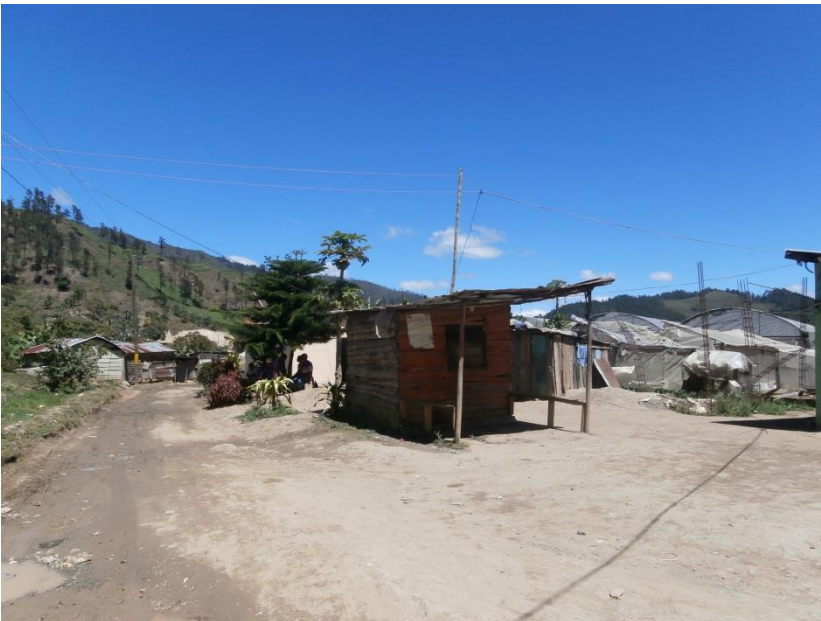
Photo 22. Grid (house connection) Arroyo Frio
