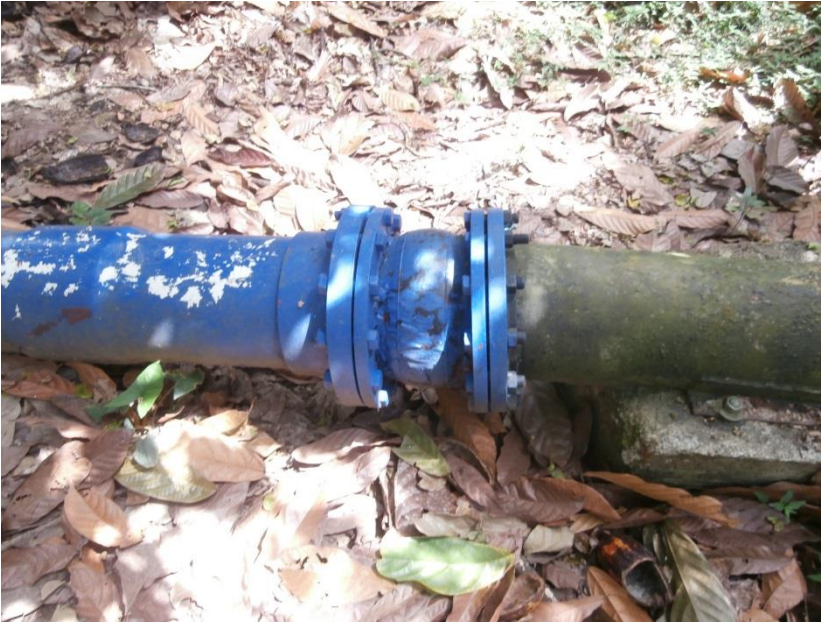
Photo 39. Joint iron-PVC pipeline Arroyo Majagua
