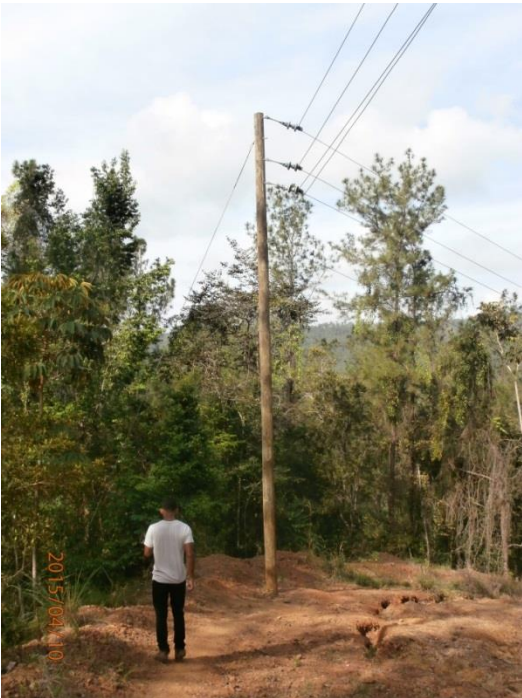
Photo 34. Grid where it is not accessible by car Montazo-Vallecito
