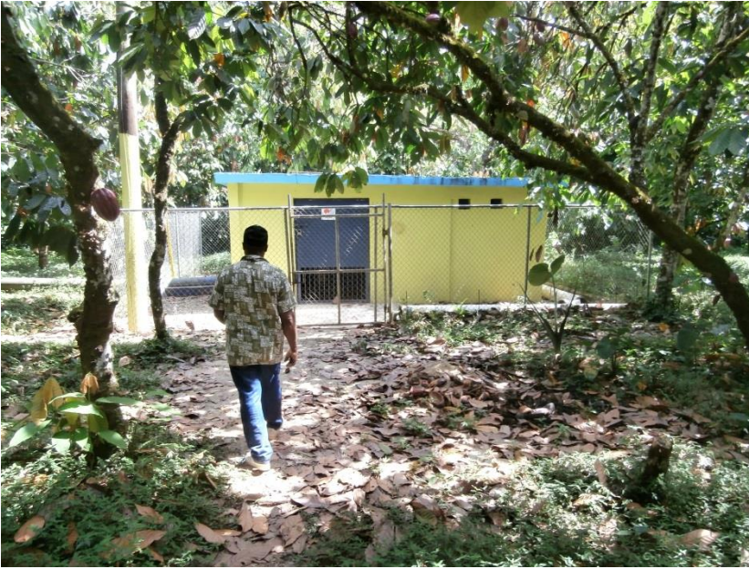
Photo 37. Power house Arroyo Majagua
