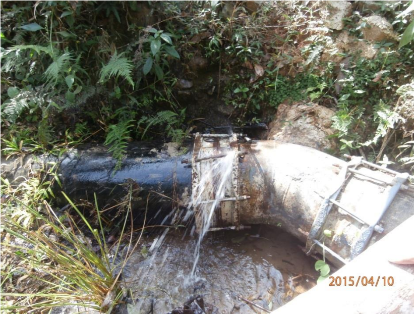
Photo 27. Joint Iron-PVC pipeline Montazo-Vallecito
