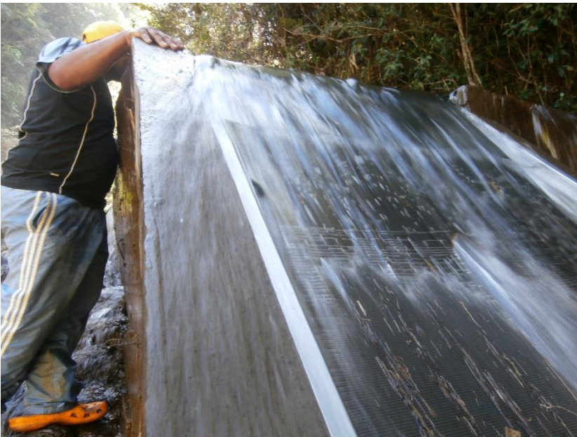
Photo 18. Grit removal Arroyo Frio
