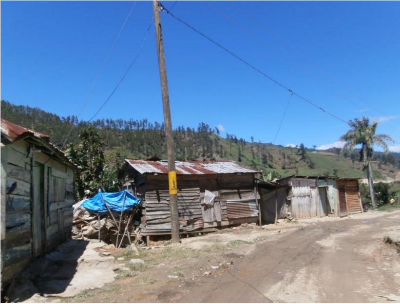
Photo 21. Grid (house connection) Arroyo Frio
