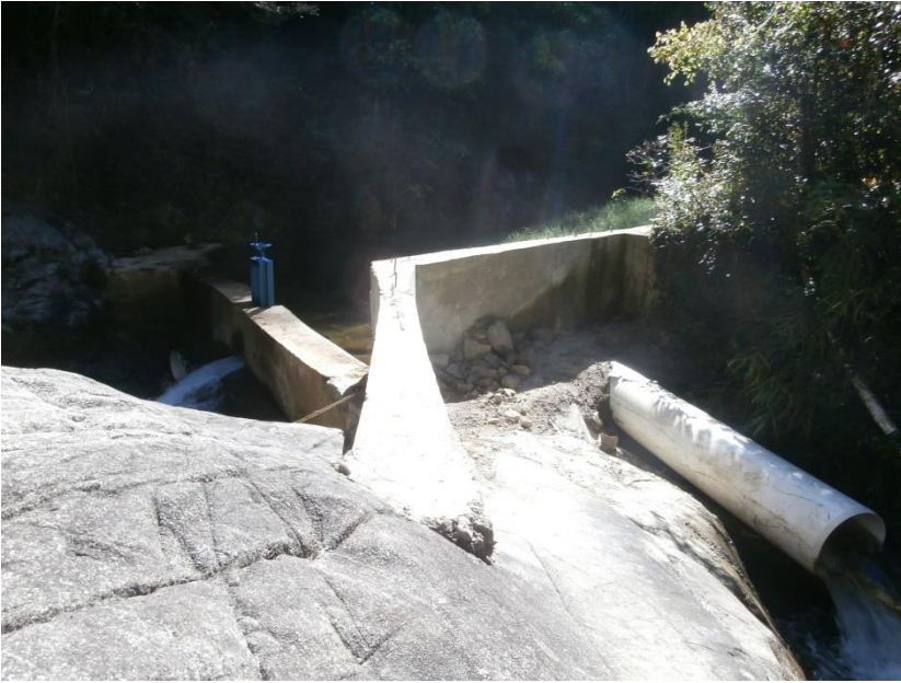
Photo 19. Water intake Arroyo Frio
