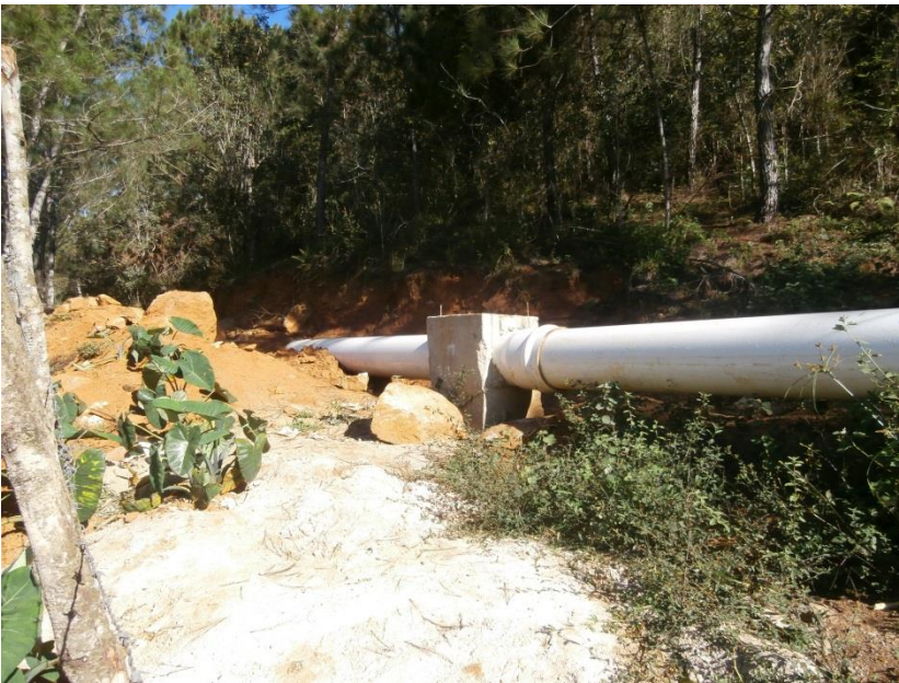
Photo 14. Columns to hold the pipe Arroyo Frio
