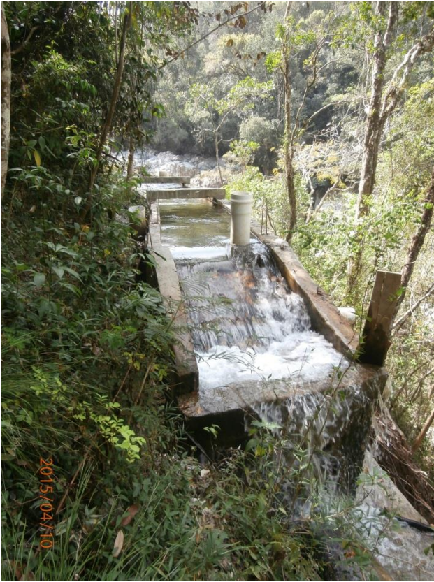
Photo 29. Grit removal (before cleaning) Montazo-Vallecito
