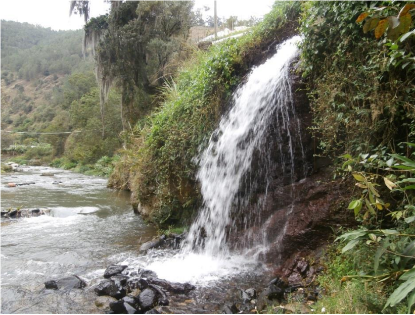
Photo 3. Water going out of the turbine Paso de la Perra
