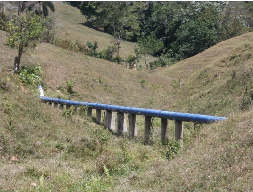
Photo 40. Columns to hold the pipe Arroyo Majagua
