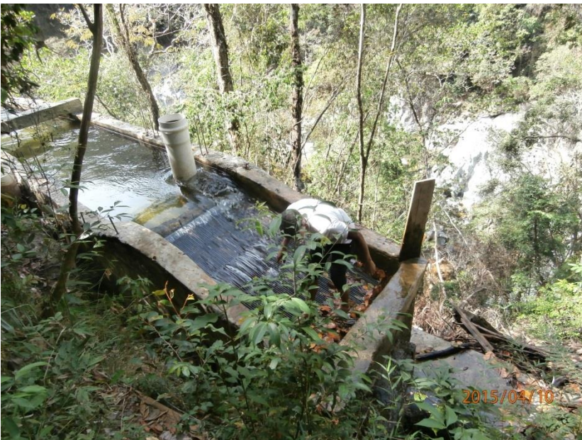
Photo 30. Grit removal (after cleaning) Montazo-Vallecito
