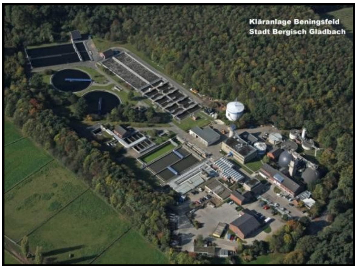
Figure 4. Wastewater treatment plant of the city of Bergisch Gladbach, Germany.
