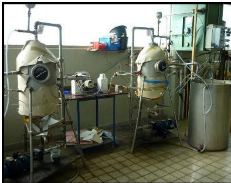
Figure 12. Set up of the pilot plant (by the author, 2014).
