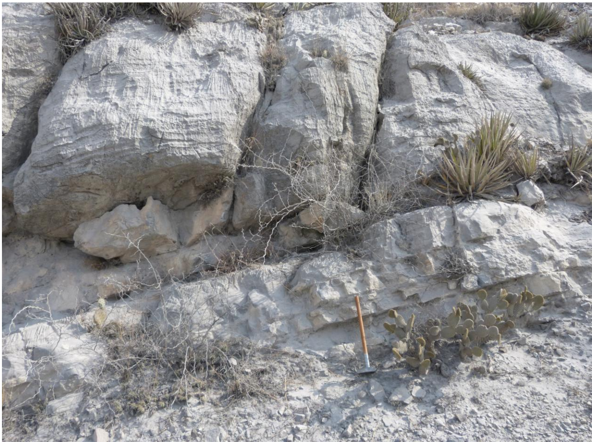
Fig. 35: The picture shows the lower part of the section Grava. The middle to thick bedded limestone is covered with dust from the quarry.
