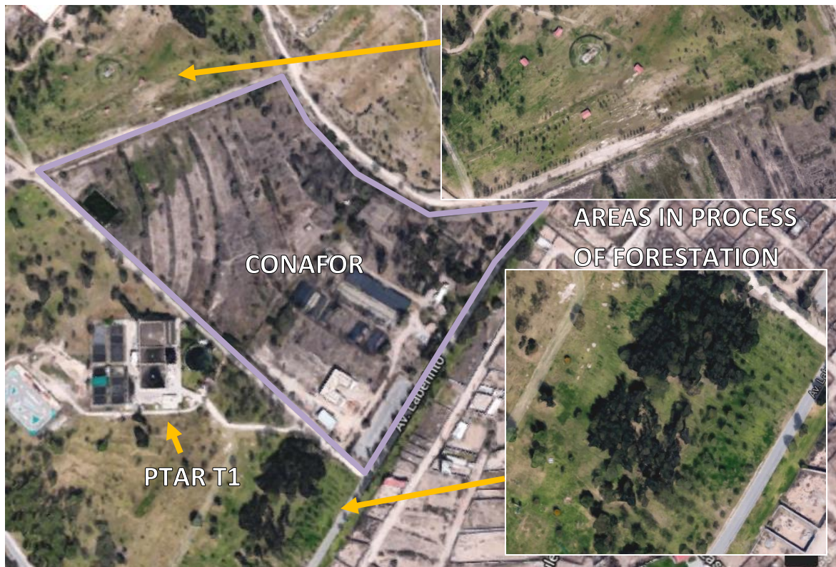
Figure 16. Plant location with respect green areas (Google/INEGI 2016).
