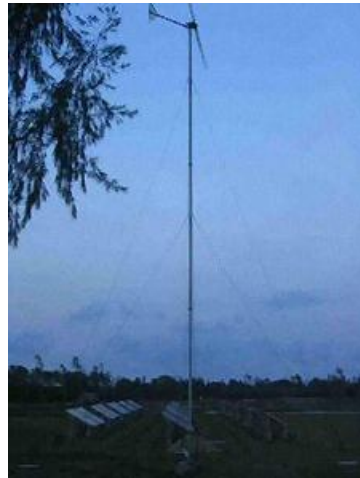
Figure 5.3-3 Hybrid Power System on Sagar Island, India, including a small-scale wind turbine and PV
