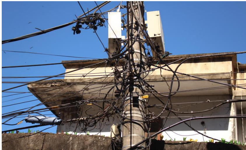
Figure 2 Electric cables in the 'Babilônia' favela, Rio de Janeiro, 2018
