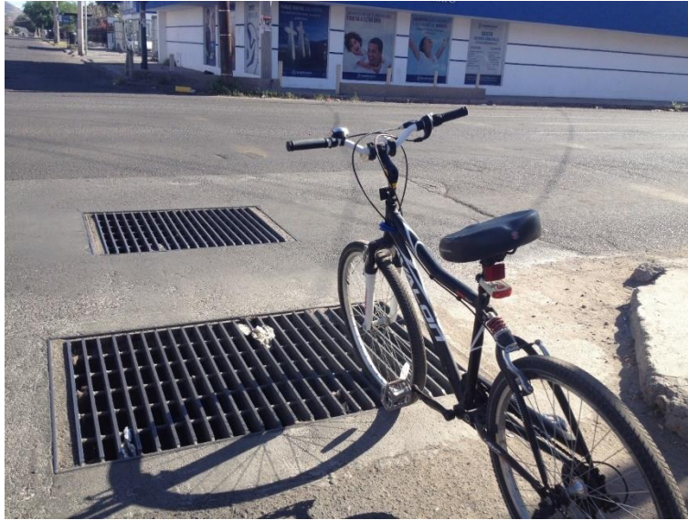
Figure 50. Rainwater drain through current bike path
