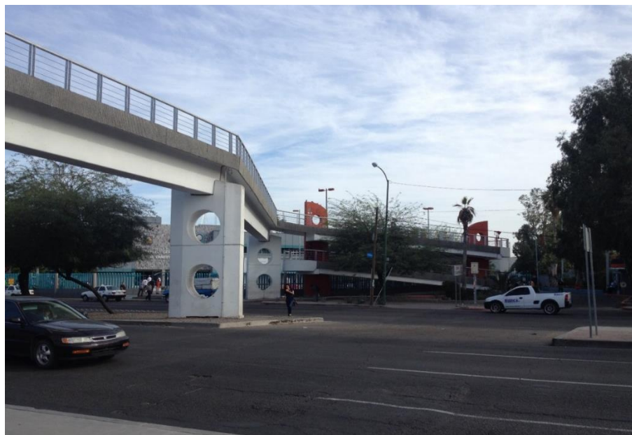
Figure 30. Overpass built in Blvd. Luis Encinas, Hermosillo
