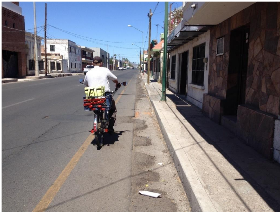
Figure 51. Bike lane isn't properly paved
